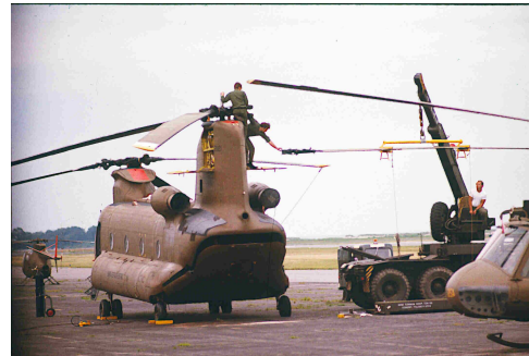
Back in the 1970's, technicians of what was the 1109 th AVCRAD replace rotor blades on the ramp. Note the other two types of whirly-birds visible.
